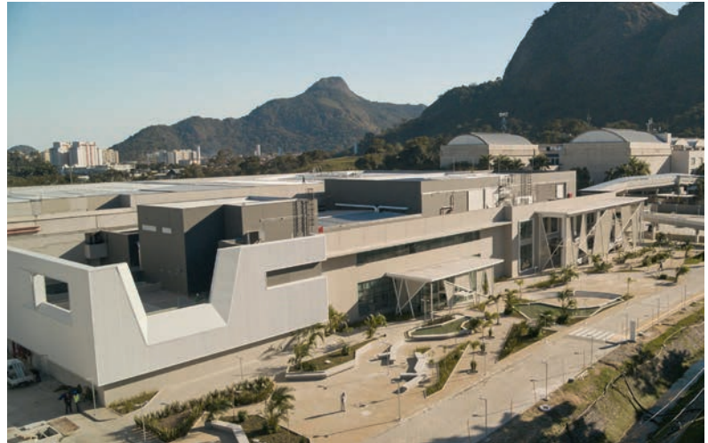
Globo's new studio complex totals 4,500 square metres
